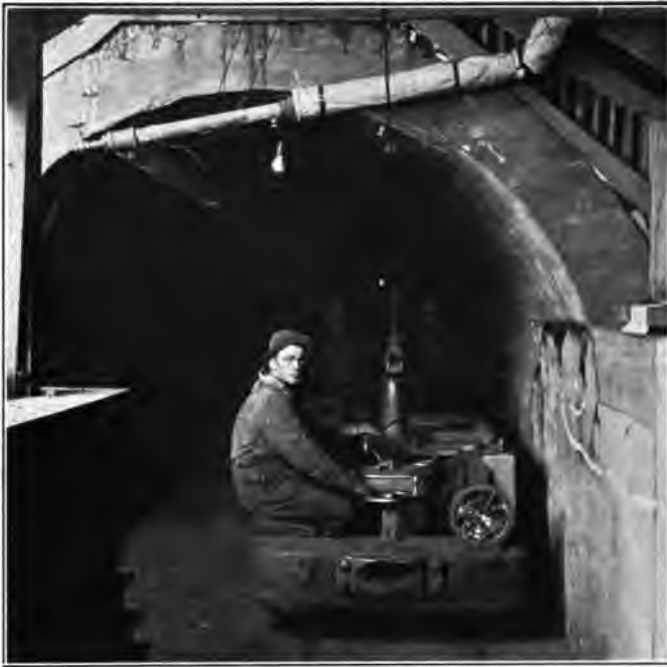
TIMBER TUNNEL NEGAUNEE MINE—USED FOR CONVEYING TIMBER FROM YARD TO CAGE BELOW COLLAR OF SHAFT
